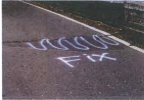
A section of the roadway has settled.
