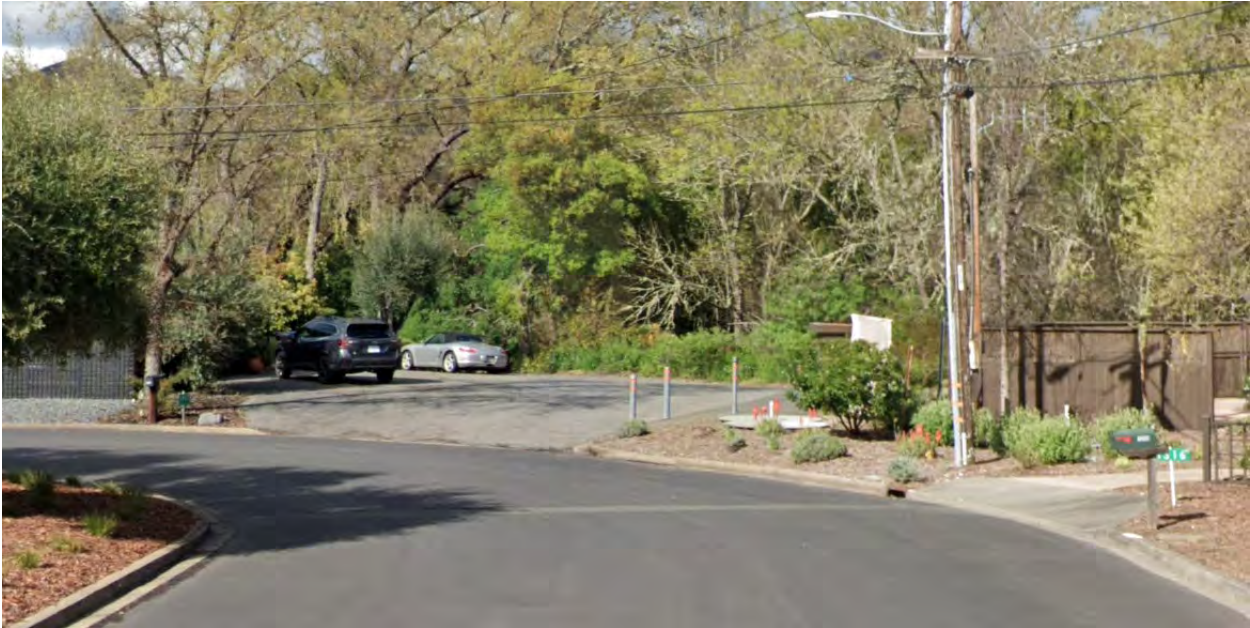
Figure 5. Oak Street - Lack of Curb Ramp and Missing Sidewalk
