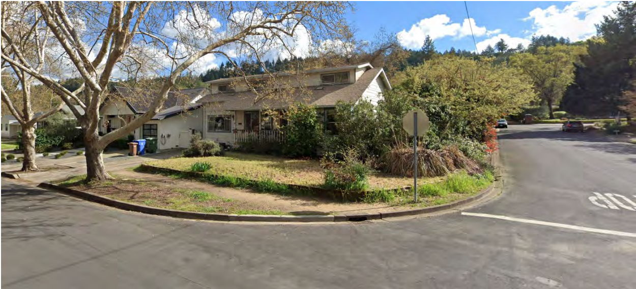
Figure 4. Cedar Street - Lack of Curb Ramp and Missing Sidewalk
