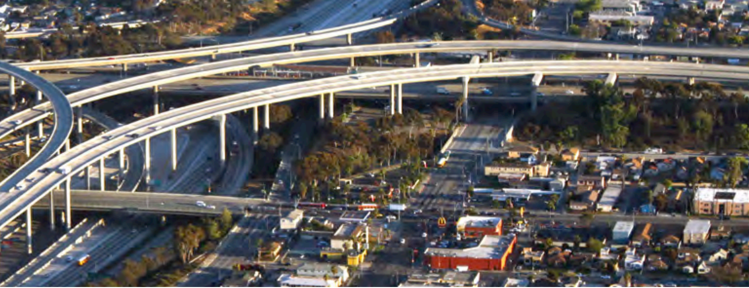
I-405, Los Angeles, CA. Built in 1961. Photo Credit: Prayitno
